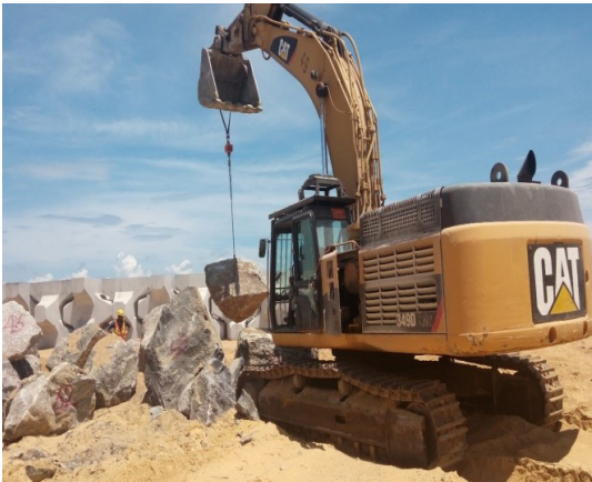
Grading test for armour rock
