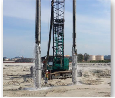
Dynamic Compaction Method
