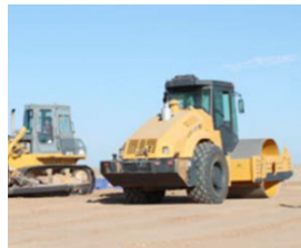
Dynamic Compaction Method
