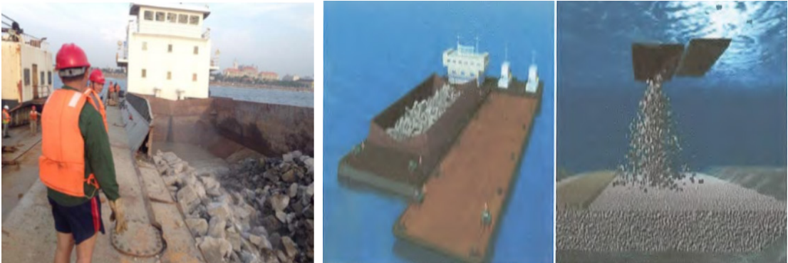
Fig 6 : Rock filling by 1000 m 3 split barge
