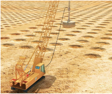
Dynamic Compaction Method
