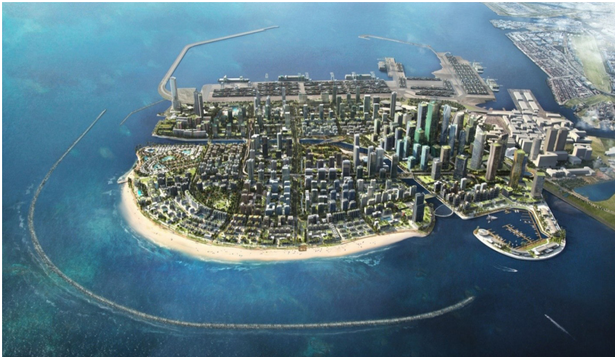
Fig 1 : Breakwater general view after completion
